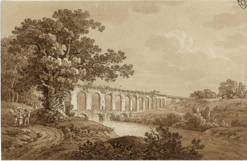
Figure 4. The partly dismantled Altväterwasserleitung in Halsbrücke, by Adrian Zingg, 1790s. The structure is captured in picturesque style even as its wooden components remain in place on the far bank and across the top. Kupferstich-Kabinett, Staatliche Kunstsammlungen Dresden, Inv.-Nr. A 131949, Photo: Herbert Boswank.
